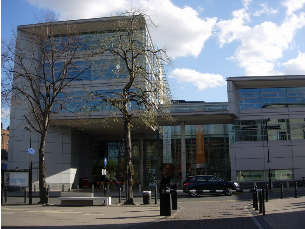
Figure 3; Site viewed from the north
