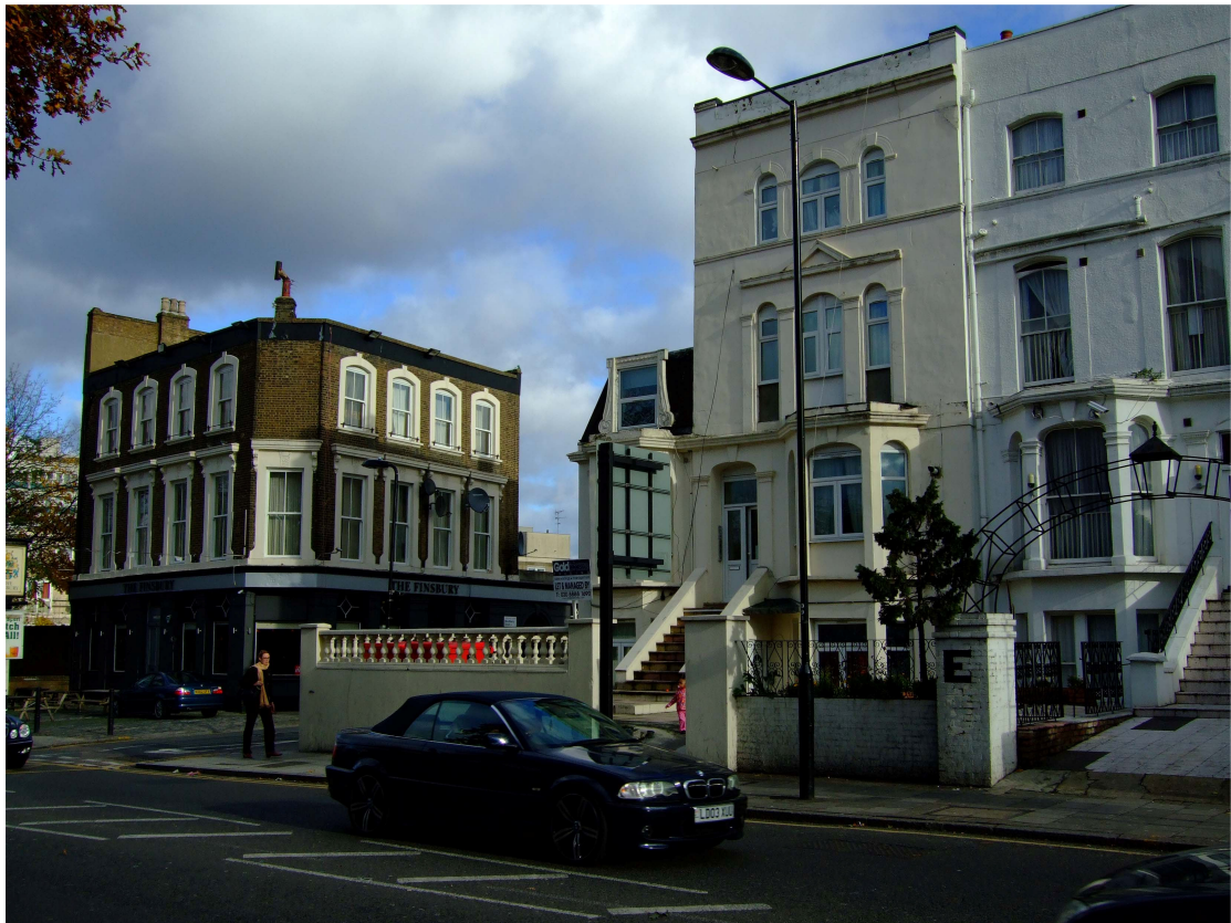
Front elevations of adjoining buildings, 332 and 336 Green Lanes
