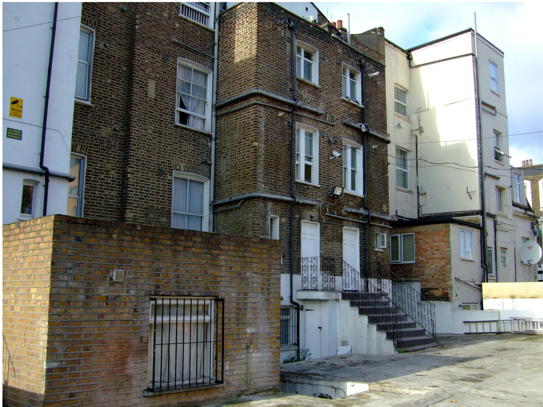
Rear of 326-330 Green Lanes
