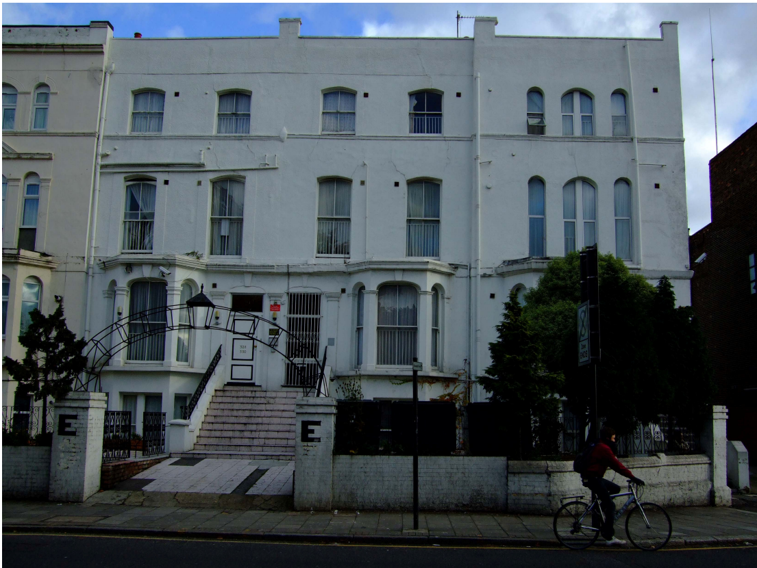
Front elevations of existing buildings at 326-330 Green Lanes
